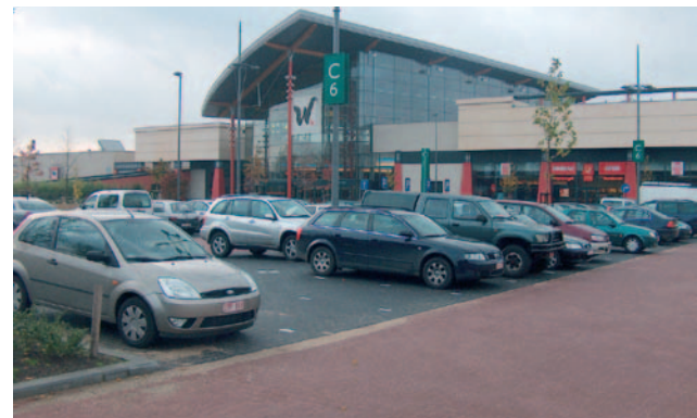
Parking pavement made with permeable paving blocks
