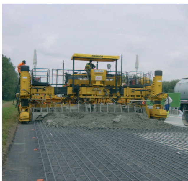
Continuously reinforced concrete
