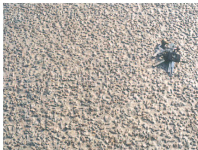
Fine exposed aggregate surface
