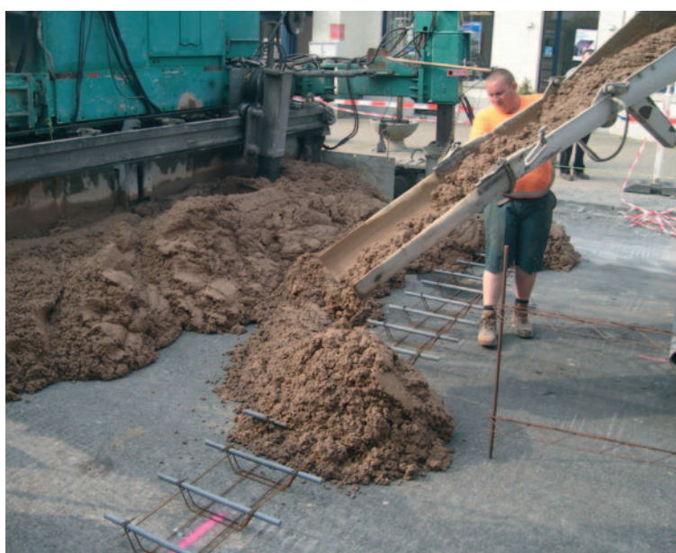
Dowelled plain concrete
