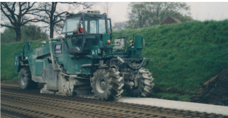
Soil treatment with cement
