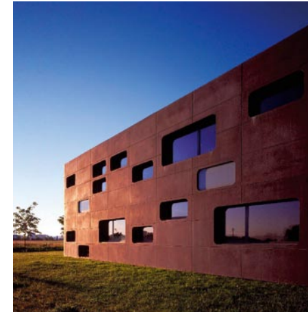
Graphical concrete techniques offer added potential for choice in facades. Wall facade in Germany. Copyright: Betonmarketing Süd, 2004 (Foto: Guido Erbring)
