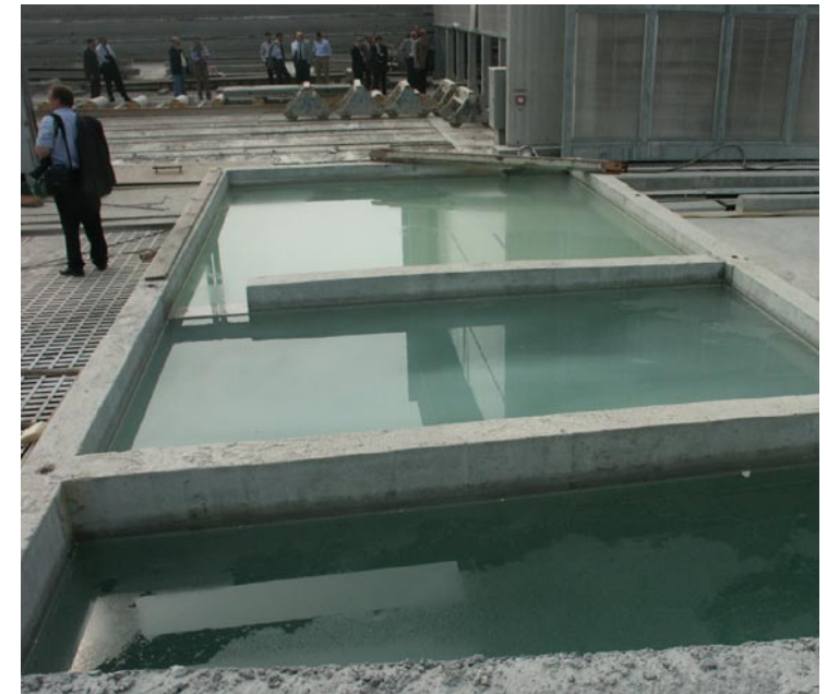
The solid material in process water in the concrete industry is allowed to settle out so the water can be recycled for concrete manufacture. Courtesy Betoni, Finland.
