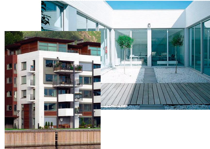
Concrete-framed buildings can be designed with a variety of appearances to blend in with the environment.
