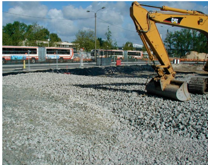
Recovered waste material and crushed waste concrete can be used in road construction. Credits: Photothèque CERIB.
